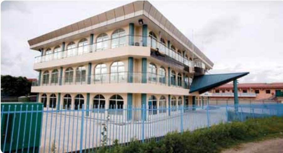
New Century 21 Building housing iPi Catering office – just prior to completion, Port Moresby
